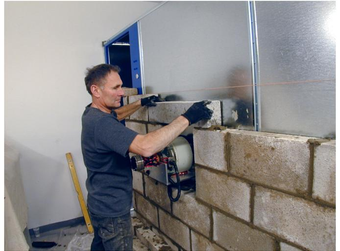
Covering the beam line end of the Faraday cage with staggered, offset blocks.
