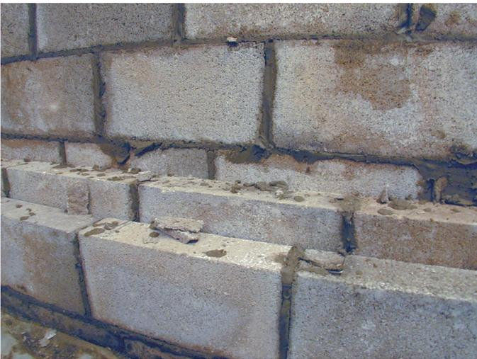
This type of construction ensures minimal radiation leakage consequences due to potential 'gaps' in the block-work.
